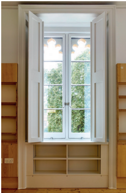
Window shutters and architraves (left) were brought forward slightly to accommodate secondary glazing, security fixings and wall insulation. Bookcases and other fittings on either side were designed to accommodate services and (right) to hide an en suite shower. All showers were located away from exterior walls to avoid contributing to the moisture load. (All photos: Tim Soar)
