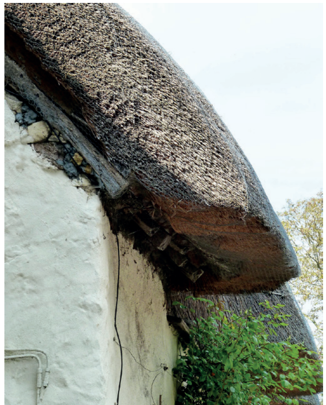
The depth of thatch shelters the wall below. If the thatch were replaced with tile or slate (as so much was) the wall becomes very vulnerable.
