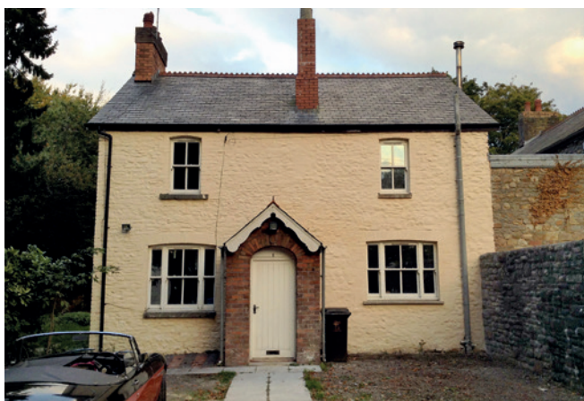
Mill Cottage on completion of repointing and lime-washing using Vivus materials
