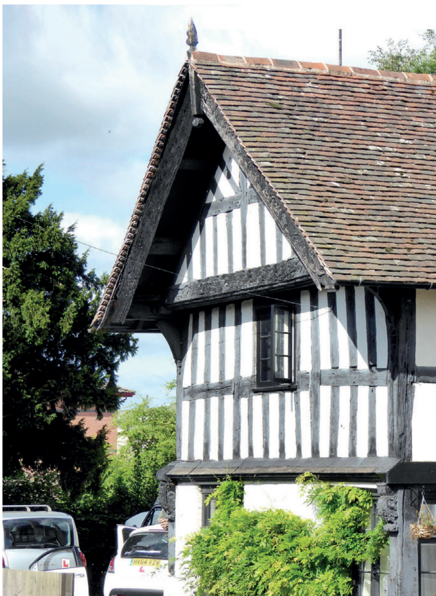
The large original verge overhangs of this historic timber-framed house protect the wall below, while an angled 'pentice' board above the ground floor window sheds water away from the wall below. (All photos: Robert Demaus)
