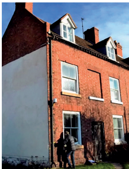
Monitoring a south-facing brick wall at Shrewsbury
