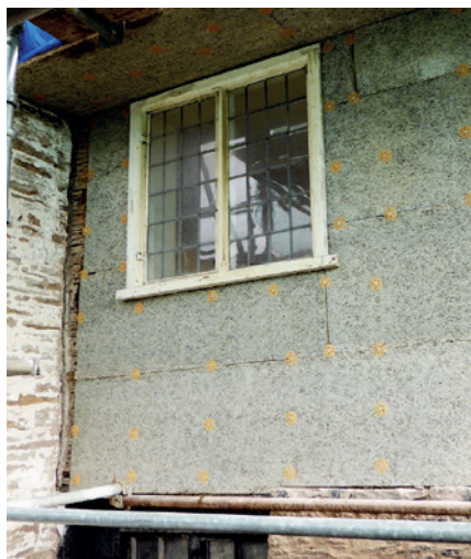
Wood-wool insulation boards ready for lime rendering
