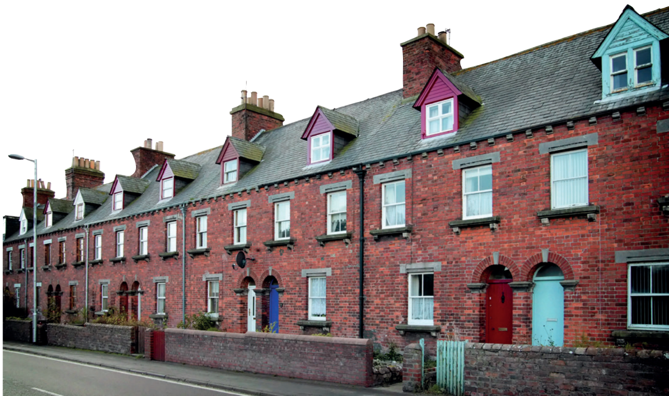
Proposals are sometimes put forward for external wall insulation to be applied intermittently to the front elevation of individual houses in a terrace, despite there being features of architectural interest. A heritage impact assessment may prevent alterations like this from happening. Aesthetics are not the only consideration under the significance umbrella, but assessing significance will inevitably mean a greater likelihood of external wall insulation being applied to plain rendered elevations than to very ornate elevations with bay windows. This terrace is somewhere between the two, which is where the more difficult decisions lie. (Photo: Historic Environment Scotland)
