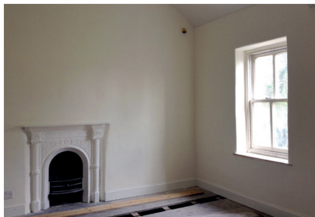
Fireplace and window details, with insulated walls, plastered and finished
