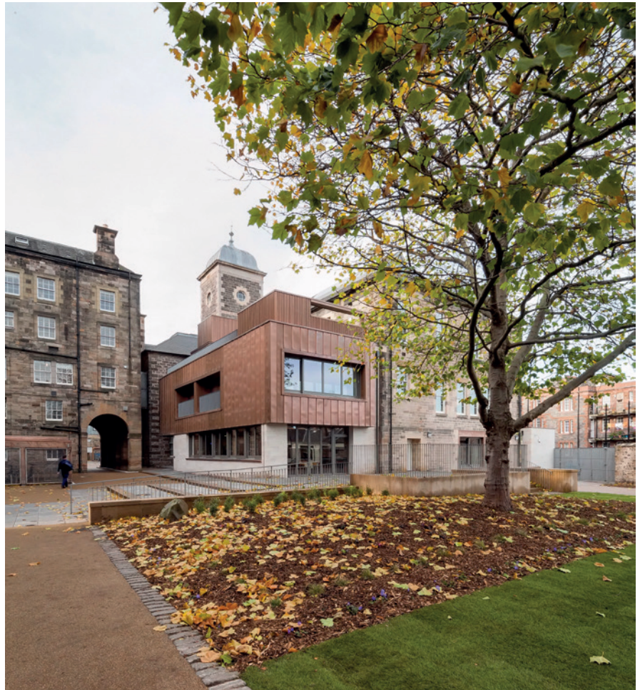
The Edinburgh Centre for Carbon Innovation, which opened in 2013, is a category A listed former school. Its refurbishment used low carbon materials including highly engineered timber and reclaimed steelwork. It is the first refurbished historic building in the UK to achieve a BREEAM 'Outstanding' rating. (Photo: Dave Morris)
