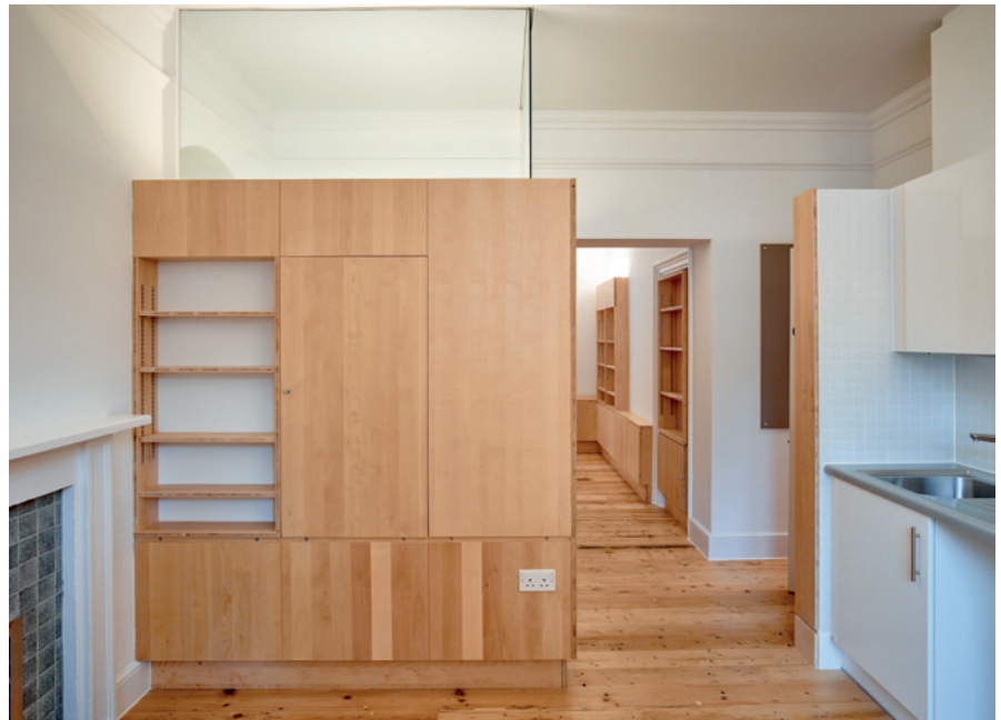
Window shutters and architraves (left) were brought forward slightly to accommodate secondary glazing, security fixings and wall insulation. Bookcases and other fittings on either side were designed to accommodate services and (right) to hide an en suite shower. All showers were located away from exterior walls to avoid contributing to the moisture load. (All photos: Tim Soar)
