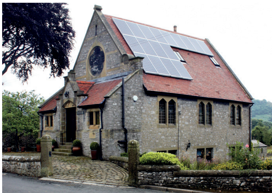
Austwick, Lancashire: house conversion. Heritage significance subsumes appearance and material fabric. In this case, whereas the material fabric has been retained by overlaying solar panels, the building's appearance has been seriously compromised. Advances are being made in the production of solar roof tiles, also shingles and slates, which protect the overall as well as detailed appearance of historic buildings but require substitution of the fabric. The heritage impact methodology outlined in this article facilitates informed and transparent decision-making in situations where choices have to be made. (All photos: Dennis Rodwell)
