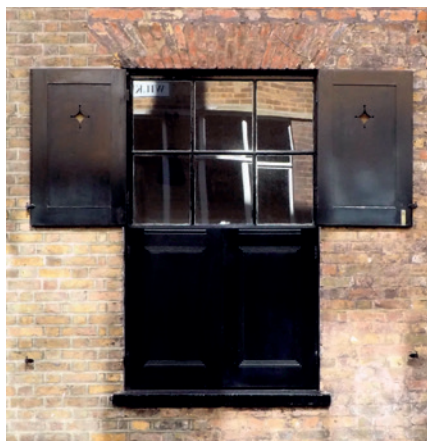
Shutters on the ground floor of a Georgian terrace in Spitalfields, London: commonly used on the continent to keep interiors shaded and ventilated during the day, here the focus was on privacy and security.
