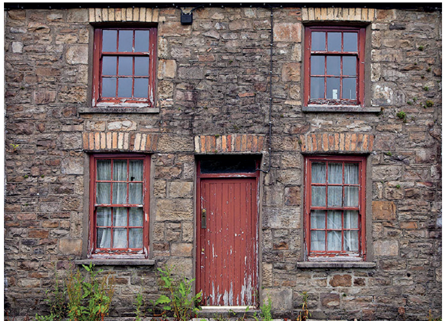
A miner's cottage in David Street, Cwmdare: analysis of the building's pathology as required under BS 7913: 2013 provided information on the effects of damp on the in situ U-value, and demonstrated that the walls were more thermally efficient than predicted. (Photos: John Edwards)
