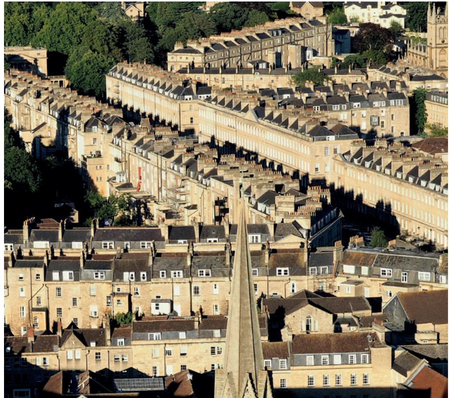
Tightly packed Georgian housing in Bath: intrinsically sustainable design with a low ratio of external envelope to interior
