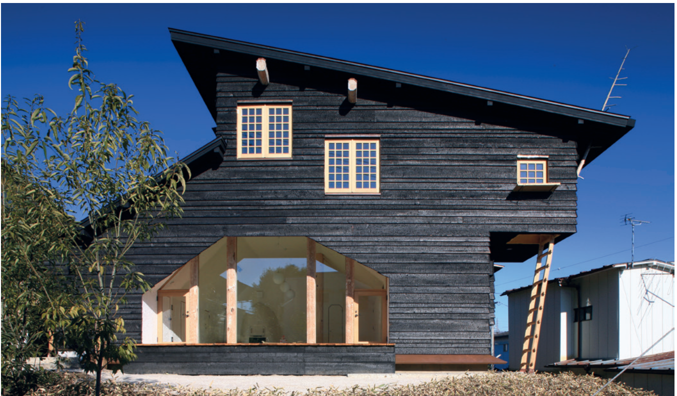
Yakisugi cladding on a house designed by Terunobu Fujimori in Utsunomiya, Tochigi Prefecture, Japan (Photo: Dana Buntrock, Flickr)
