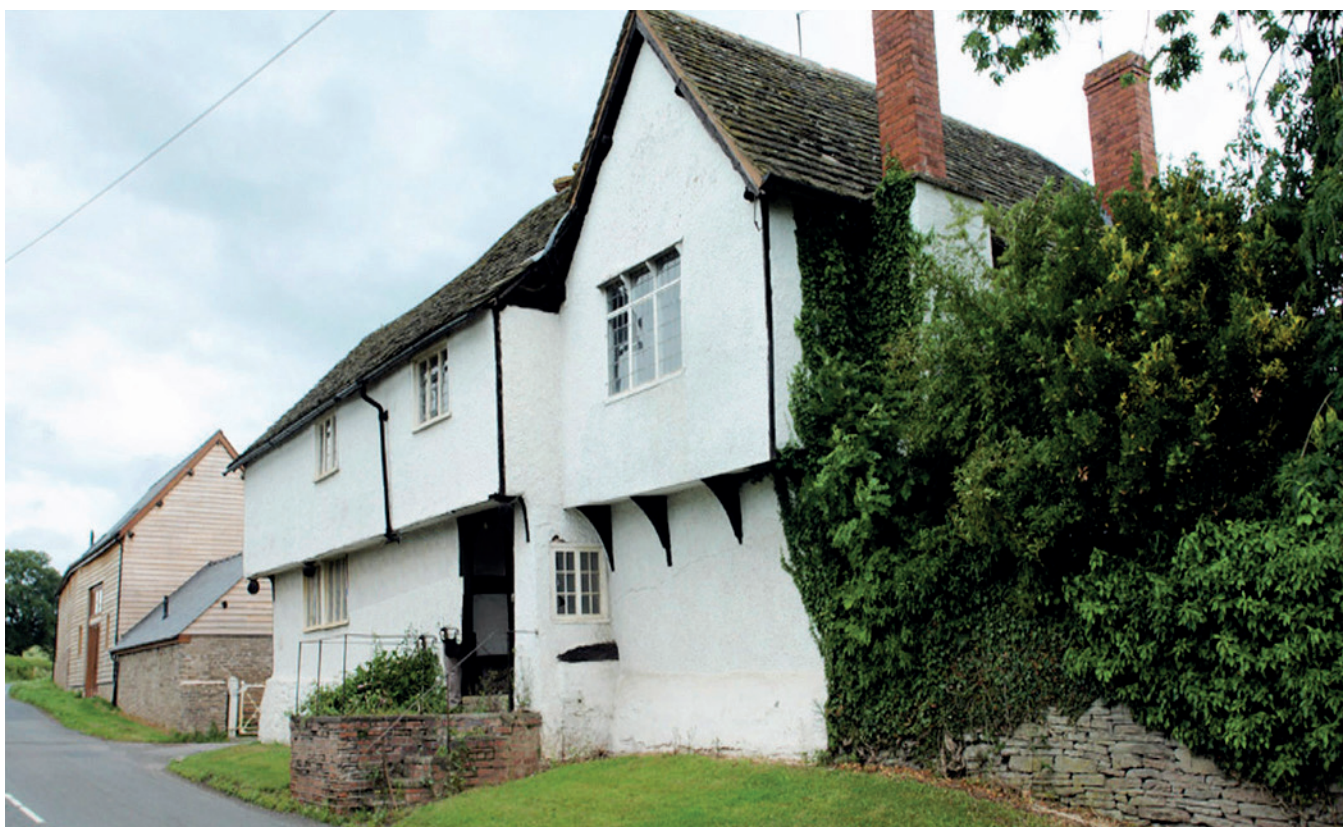
Historically, many timber-framed buildings were rendered to improve their weather-tightness. Some of the visible render is lime-based and probably early 19th century, other sections have been replaced with a cementitious render in the 20th century.
