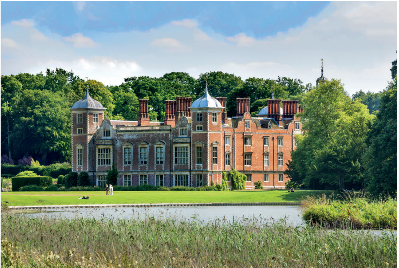
Blickling Hall in Norfolk, where the National Trust recently installed a 200kW lake source heat pump to heat the main hall
