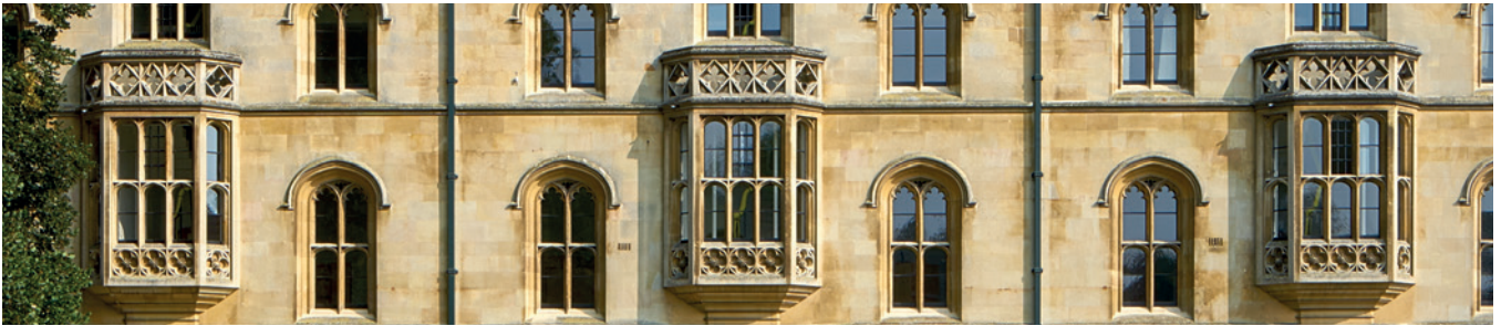
Detail of the fine riverside elevation of New Court, Trinity College, completed in 1825 and now listed Grade I (Photo: Tim Soar)
