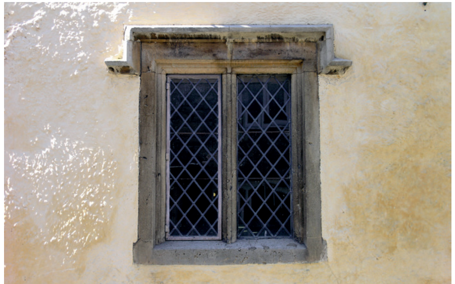
A traditional roughcast lime render on a solid masonry wall
