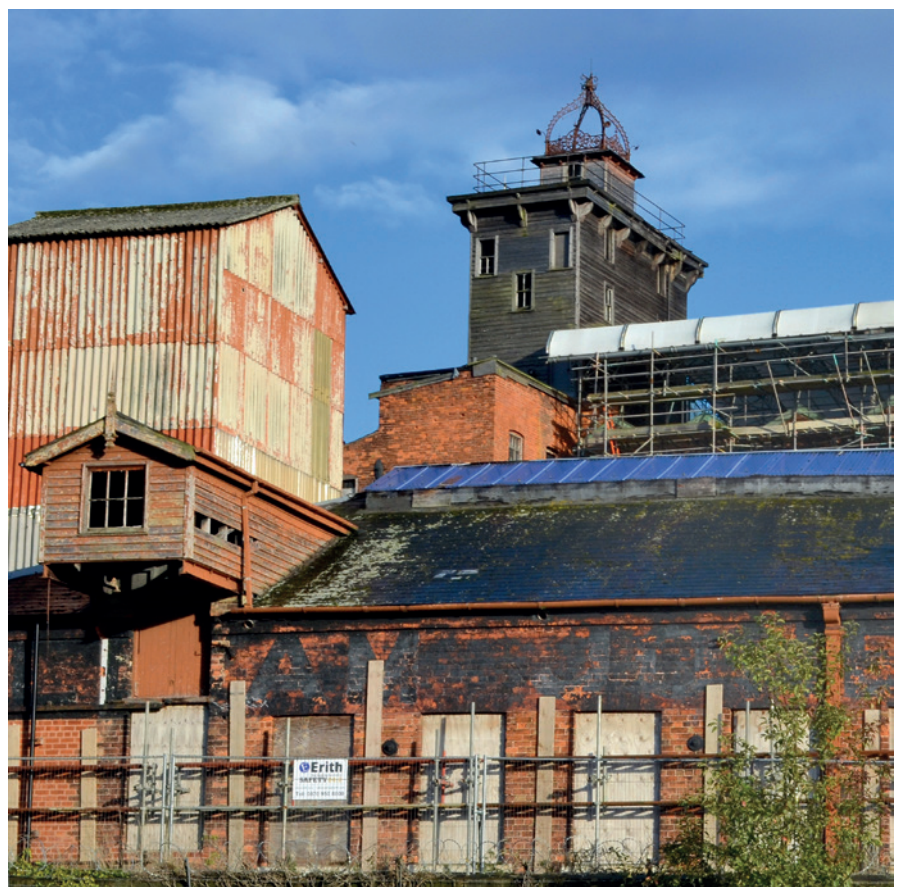
Shrewsbury Flaxmill Maltings (Grade I, 1797), where Historic England is assessing the effects of internal wall insulation on the hygrothermal behaviour of brickwork (Photo: Jonathan Taylor, all other images: Iain McCaig/Historic England)
